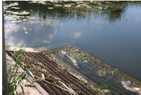
Hwy C Camp Lake Outlet box dam
