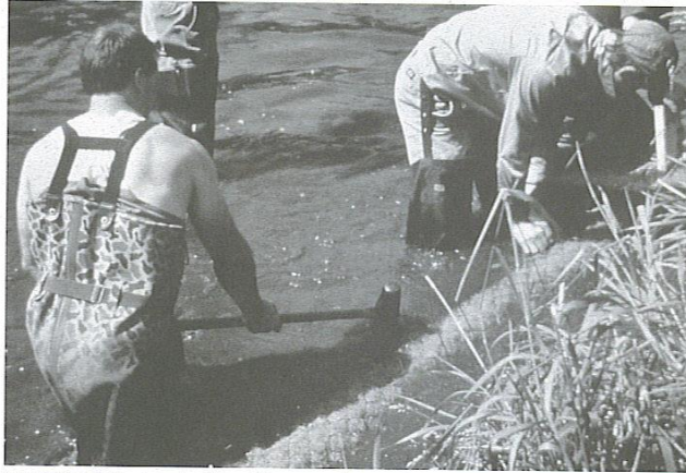
Installation of fiber logs by Natural Resources Conservation Service (NRCS) employees.
