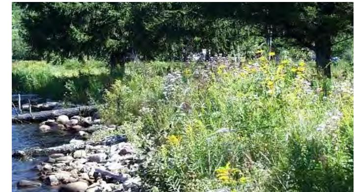
FIGURE 10: VEGETATED ROCK RIPRAP TOE
