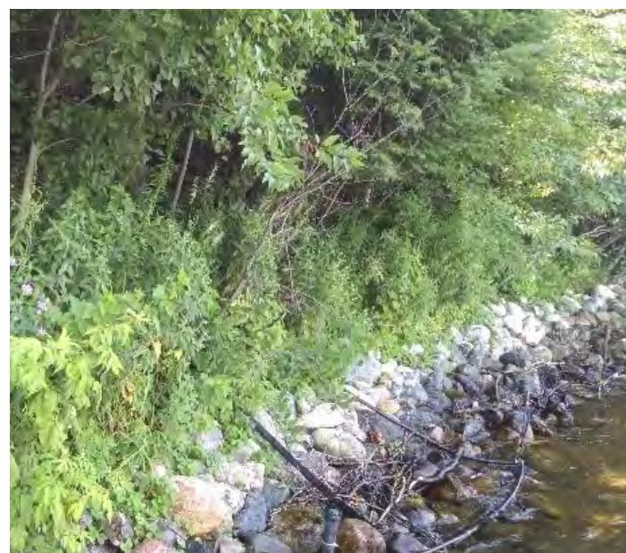
**FIGURE 12: ROCK RIPRAP TOE WITH UPLAND VEGETATED GEOGRID LIFTS**
