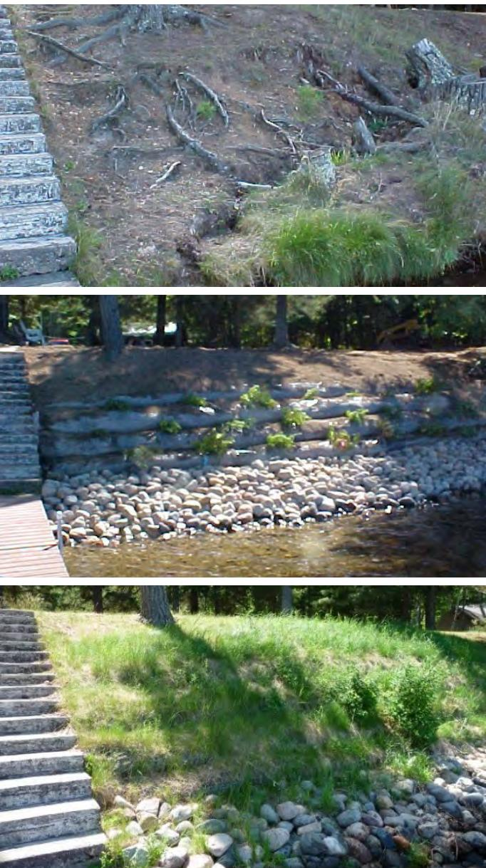
**FIGURE 13: SYNTHETIC ENGINEERED MATTING**
